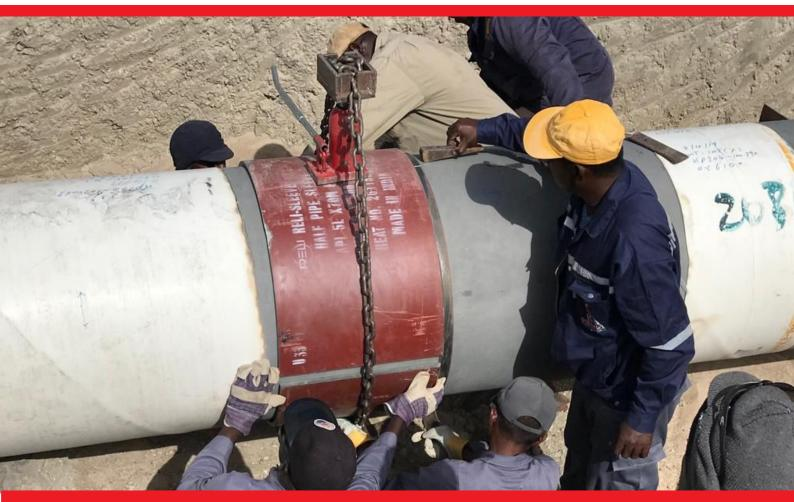
Half Pipe Sleeve Half Sole Repair Sleeve
